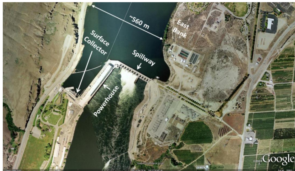
Figure 3.1 Dam 1 aerial photo.
